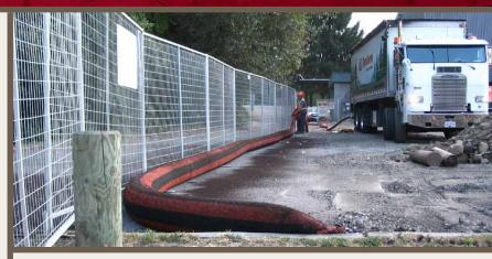
Vegetated filter socks can be left in place to provide long-term filtration of stormwater as a post-construction best management practice (BMP). The vegetation grows into the slope, further anchoring the filter sock. Vegetated socks can also be used for streambank restoration and living retaining walls.
