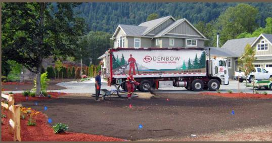
Hydroseeding = Topical application of a mix of seed, fertilizer and tackifier. The slurry is sprayed evenly over disturbed soil. Vegetation establishment depends on moisture availability (rainfall) and the nutrients in the site soil. Hydroseeding is recommended if the site soil is nutritious and already provides a good growing medium for the applied seed.
