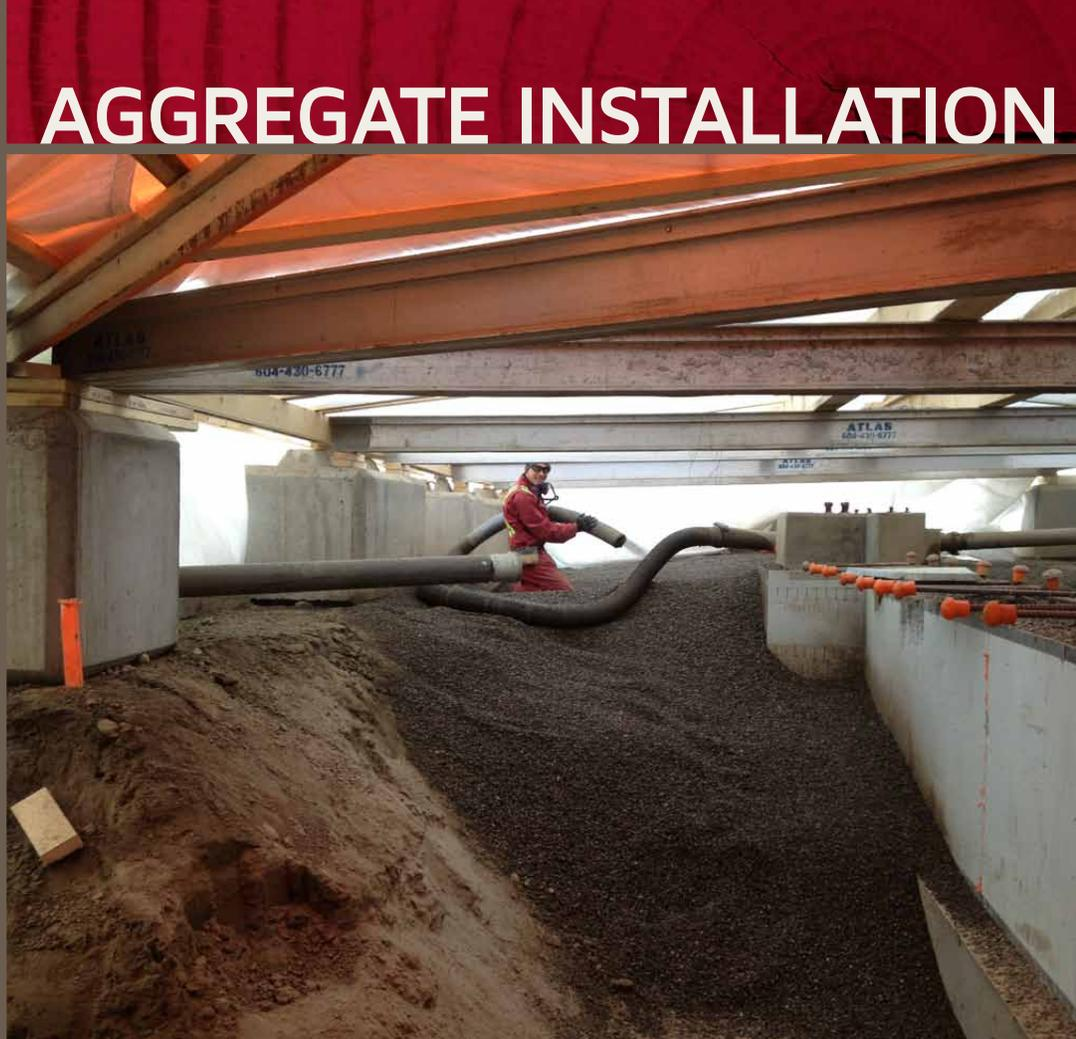
Placing aggregate pneumatically is efficient as all materials are placed exactly where required. Improve efficiency on your job sites by installing rock in hard to reach locations, in environmentally sensitive areas, and areas inaccessible by conventional equipment.
