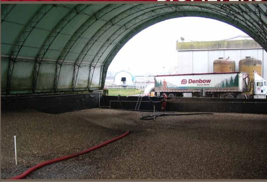
When applied to air filtration and purification, biofilters use microorganisms to remove air pollution. The air flows through a packed bed and the pollutant transfers into a thin biofilm on the surface of the packing material.
