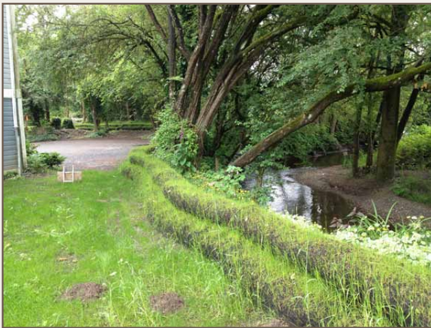
The EnviroDyke was Terraseeded™ with reclamation seed which germinates and grows to establish vegetation; the dyke becomes part of the natural landscape.
