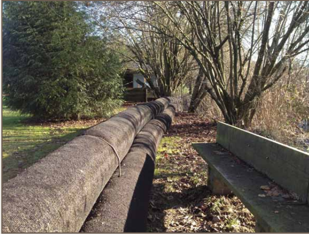
EnviroDyke installed into riparian area - 280 linear meters of EnviroDyke.
