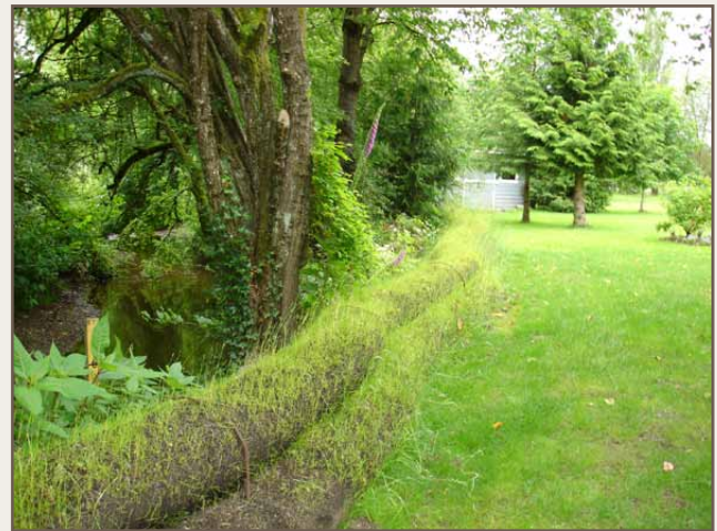
The EnviroDyke was Terraseeded™ with reclamation seed which germinates and grows to establish vegetation; the dyke becomes part of the natural landscape.
