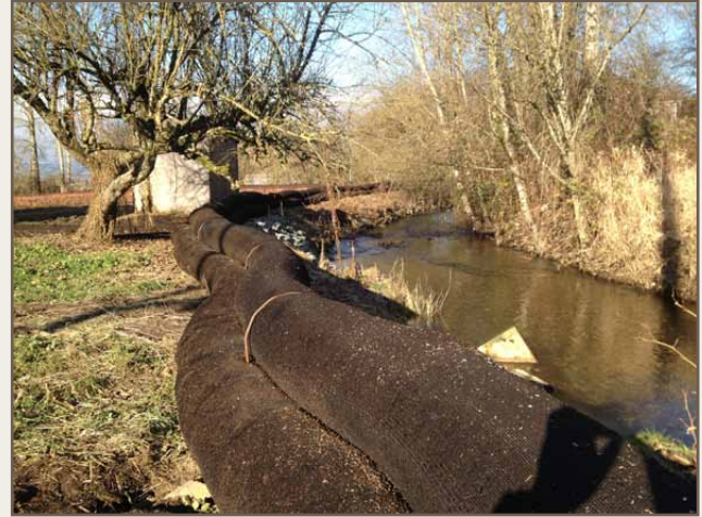
EnviroDyke installed into riparian area - 280 linear meters of EnviroDyke.
